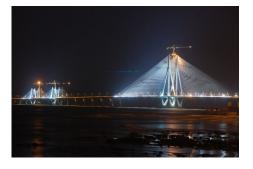
The length of the bridge is 63 times the height of the Qutub Minar in Delhi. Each cable can take a weight of 900 tons. The height of the cablestayed tower is 126m, which is equal to a 43-storey tower.
