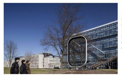
It may look like a giant airplane window strung with Venetian blinds, but this structure, designed by Dutch architecture firm Mecanoo and installed at the Delft University of Technology this month, is a model of a machine that would convert wind to energy without any moving parts.
